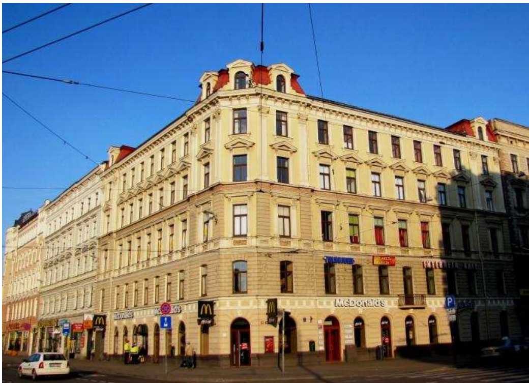
Commercial & office building – Merkela Street, Riga, Latvia
