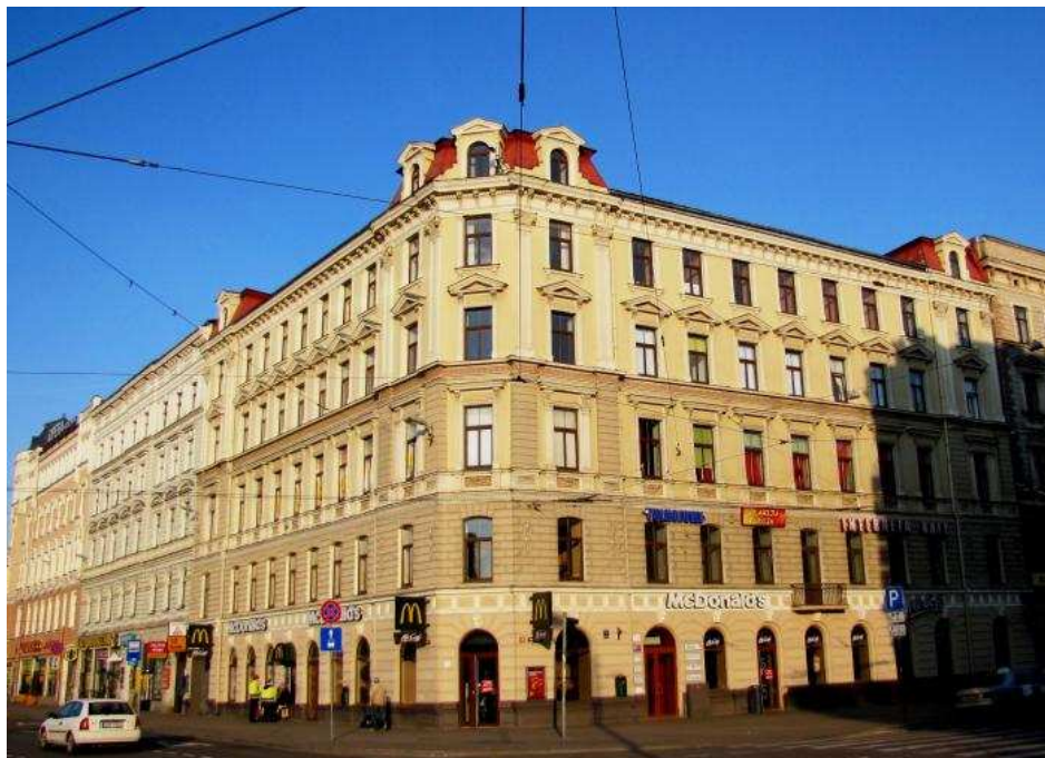
Commercial & office building – Merkela Street, Riga, Latvia
